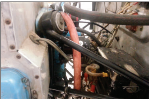
What a mess! Numerous places where wires are improperly secured and chafing. Primer lines are rubbing on engine mount. Engine has no oil filter installed, only a pressure screen.
